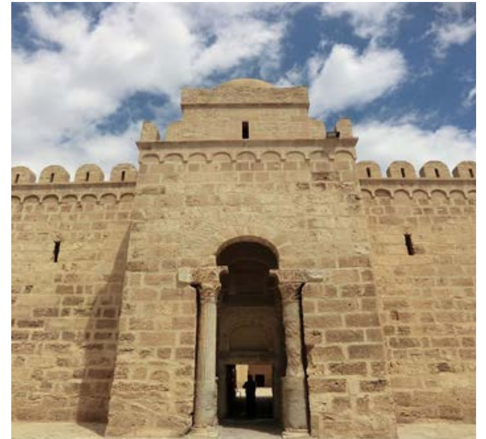
Monumental Entrance Portal at the Ribat of Sousse, flanked by two reused columns. IX century A.D
